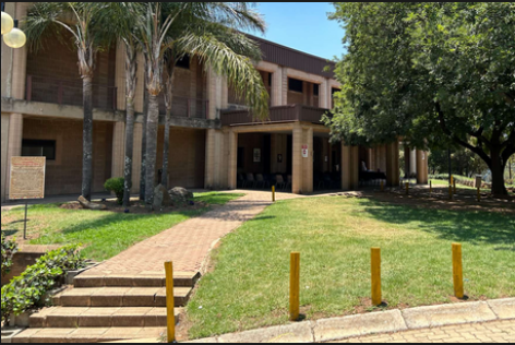
RAC exterior before
